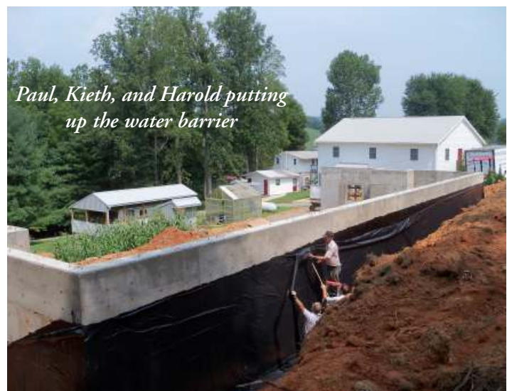
Basement walls going up
